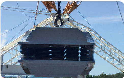
Fig. 3 Lifting of spring element with eye bolt
