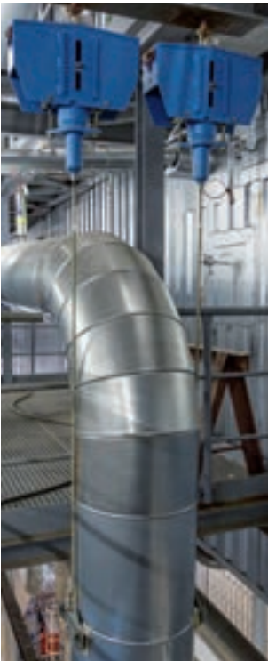
Constant hanger in a coal-fired power station
