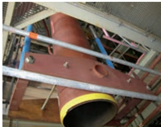
Type 34 with snubbers and position-securing devices
