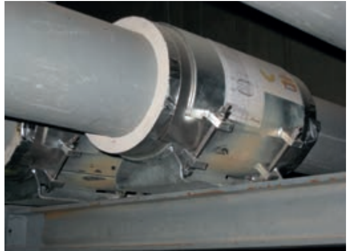
Cryogenic clamp base type 56
