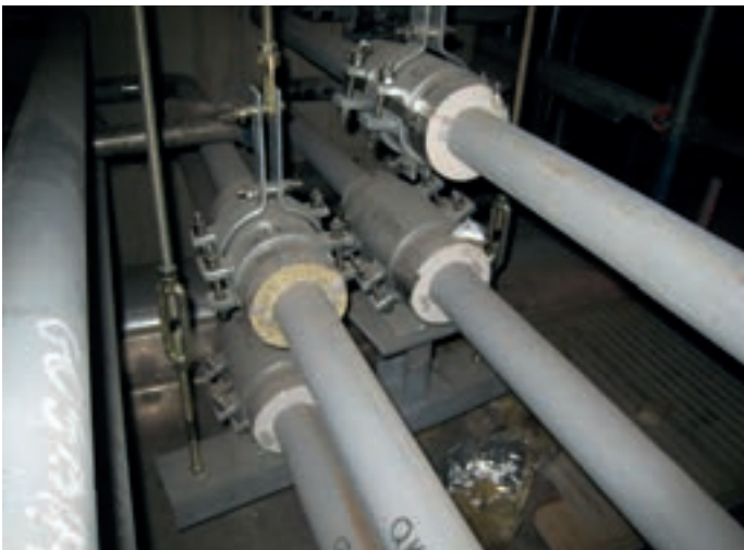
Pipes held in position with cryogenic supports
