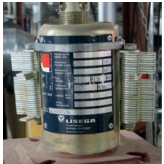
Type 29 with blocking devices attached
