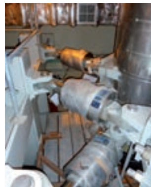
Securing pipe systems with snubbers type 30
