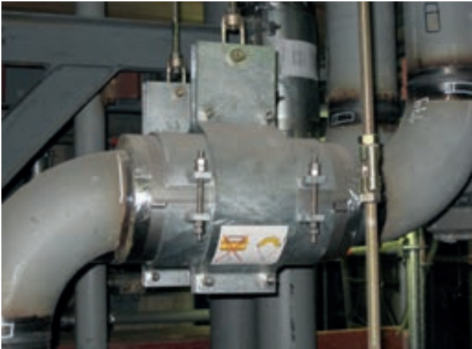
Suspension with cryogenic pipe clamps
