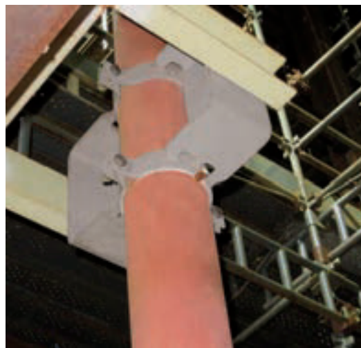
Pipe bearing (type 49 ... G2P)
