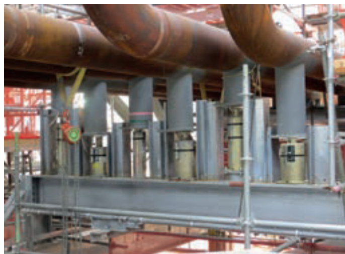
Type 58 stanchions as guides for horizontally running pipe system with type 29 spring support
