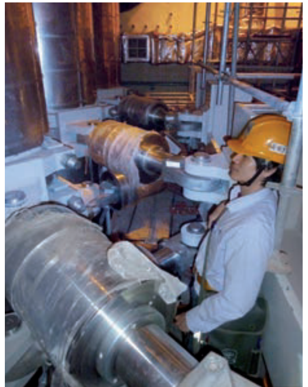
Commissioning of type 30
