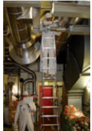
Visual inspection of snubbers
