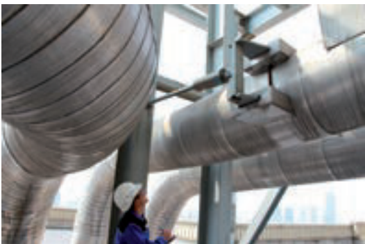
Inspection of supports at the plant
