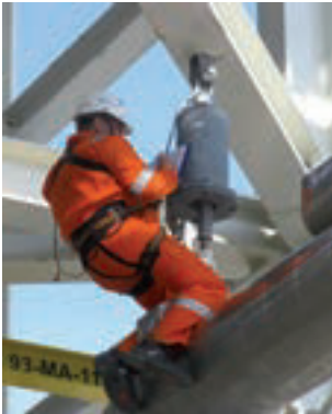
Controlling a pipe support
