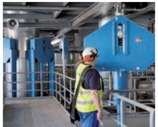
Installation inspection of a constant hanger
