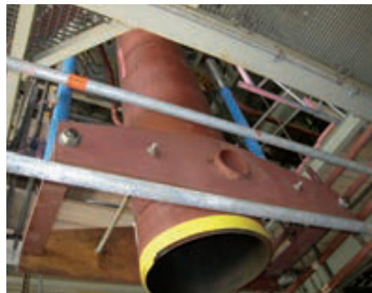
Type 34 with snubbers and position-securing devices
