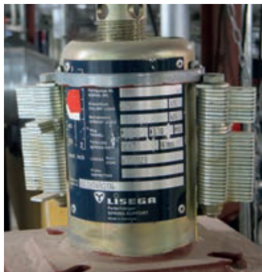
Type 29 with blocking devices attached
