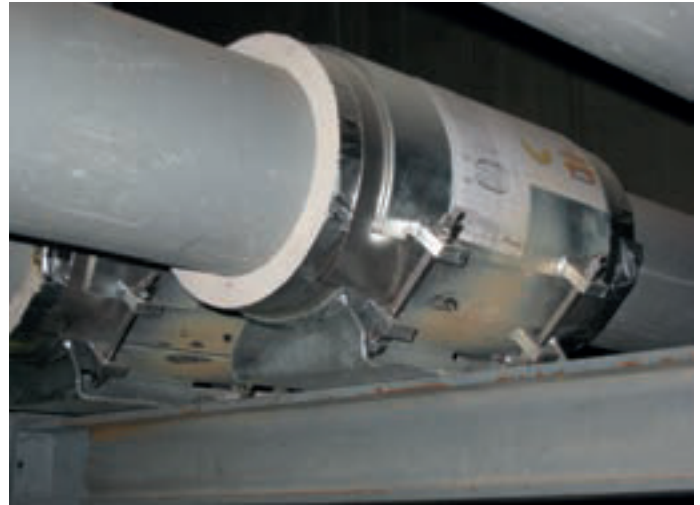
Cryogenic clamp base type 56
