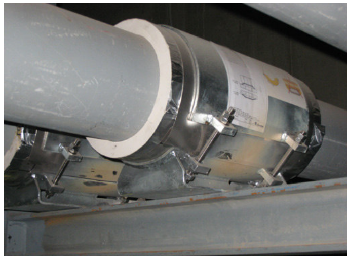
Cryogenic clamp base type 56
