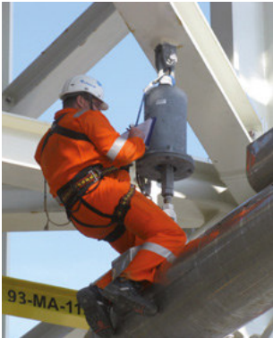
Controlling a pipe support
