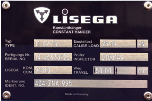
Name plate with stamped operating data
