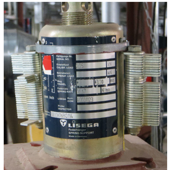
Type 29 with blocking devices attached
