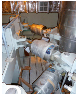
Securing pipe systems with snubbers type 30
