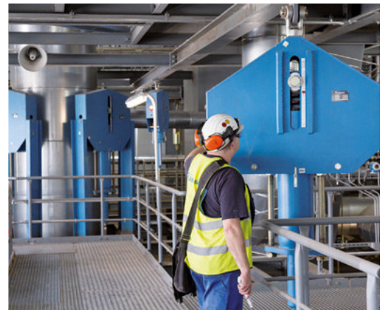
Installation inspection of a constant hanger
