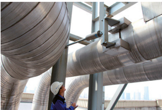
Inspection of supports at the plant
