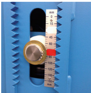
Travel scale with cold/hot marking
