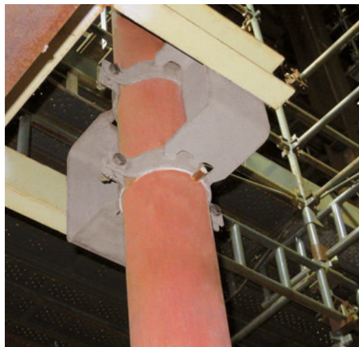
Pipe bearing (type 49 ... G2P)
