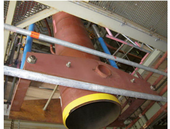
Type 34 with snubbers and position-securing devices
