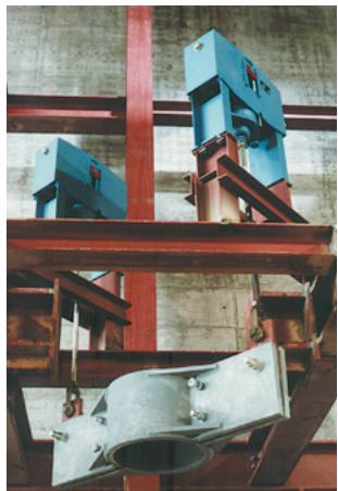
Support for a vertical pipe section with special design type 45
