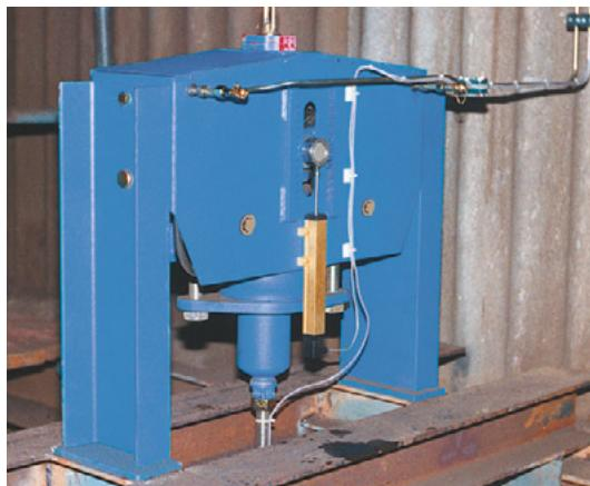
In standard cases, the temperature of the pipe system to be supported is used as a control parameter. The temperature in each case is transformed electronically into the corresponding travel position. In the theoretical / actual comparison procedure, the control ensures a regulated approach to the actual vertical elevation position.
