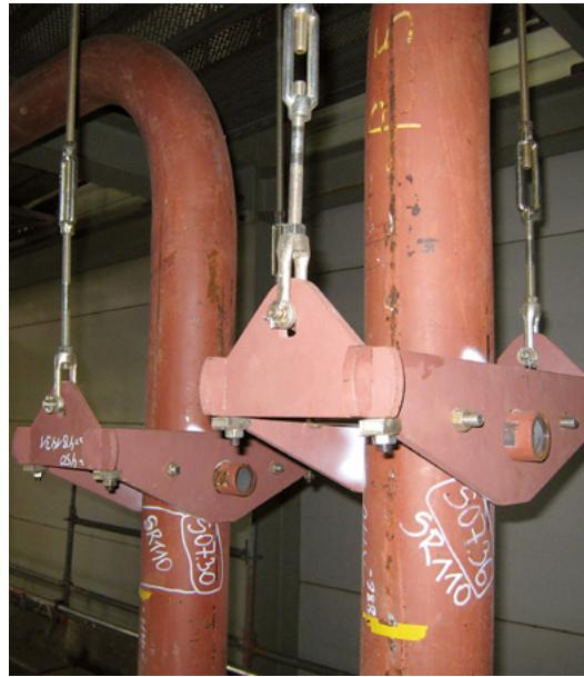
These standardized components form an integral part of the LISEGA modular system, so load and connection compatibility are correspondingly assured.
