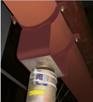
Other fields of application for LISEGA slide plates are uses where heavy loads must be moved horizontally. By using slide plates the force required for movement can be reduced by as much as 60%. The use of slide plates has a favorable effect on the whole pipe system layout.
