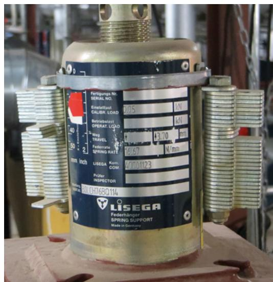
*Type 29 with blocking devices attached*
