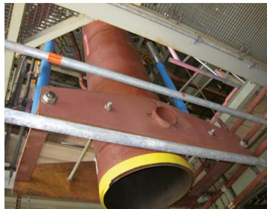
Type 34 with snubbers and position-securing devices
