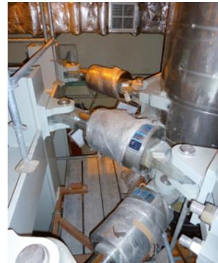
*Securing pipe systems with snubbers type 30*
