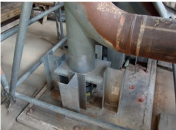
Type 58 stanchion for pipe elbows as stop free of moments in X-Y direction with type 29 spring support
