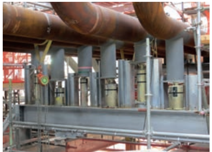
Type 58 stanchions as guides for horizontally running pipe system with type 29 spring support
