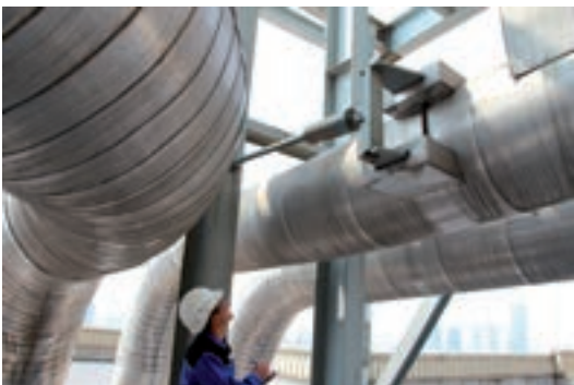
Inspection of supports at the plant
