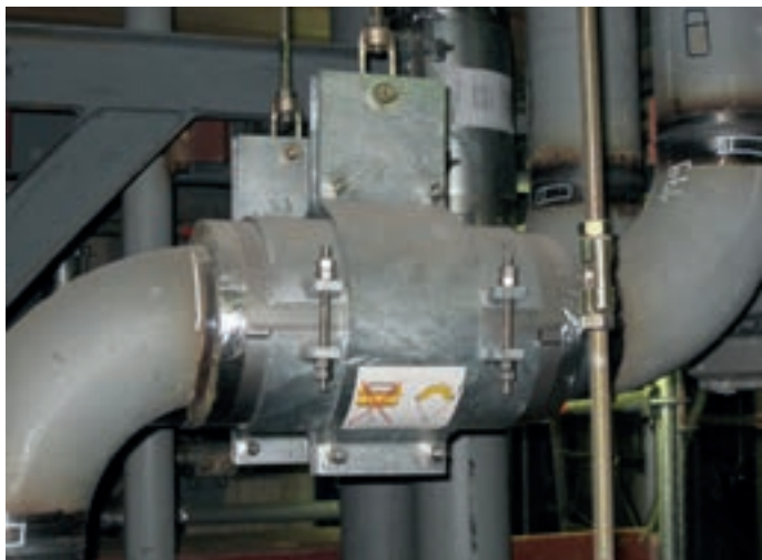
Suspension with cryogenic pipe clamps
