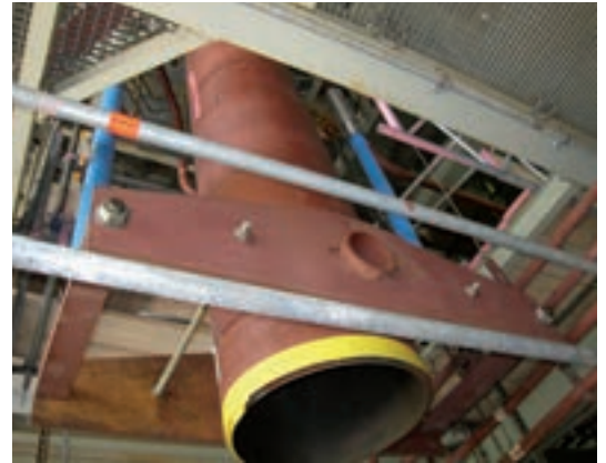
Type 34 with snubbers and position-securing devices
