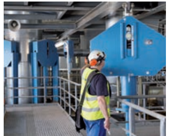
Installation inspection of a constant hanger
