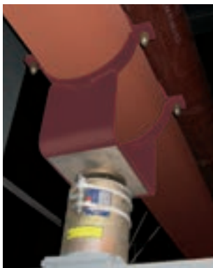
Stainless steel slide plate under clamp base type 49, high temperature slide plate and spring support type 29
