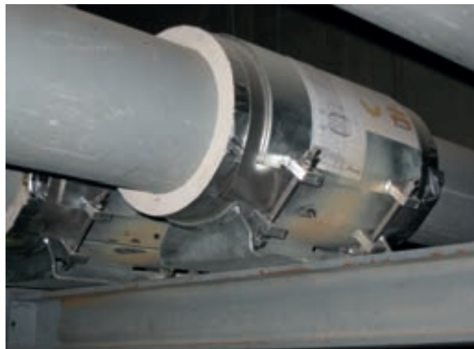
Cryogenic clamp base type 56
