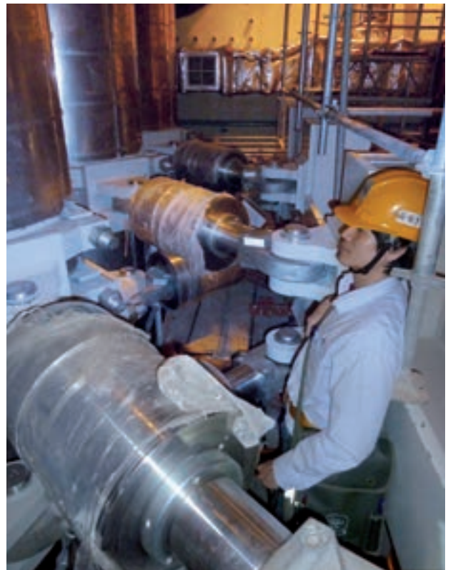
Commissioning of type 30
