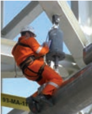
Controlling a pipe support
