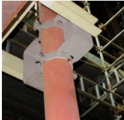
Pipe bearing (type 49 ... G2P)
