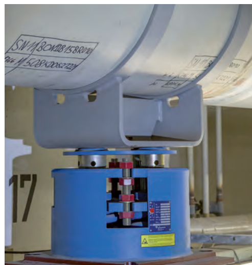
Clamp base type 49 and spring support type 28 with slide plates
