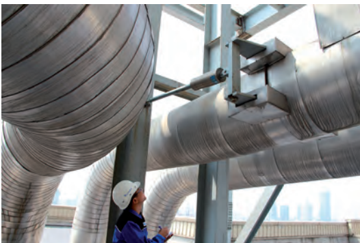
Inspection of supports at the plant
