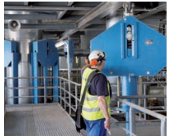
Installation inspection of a constant hanger
