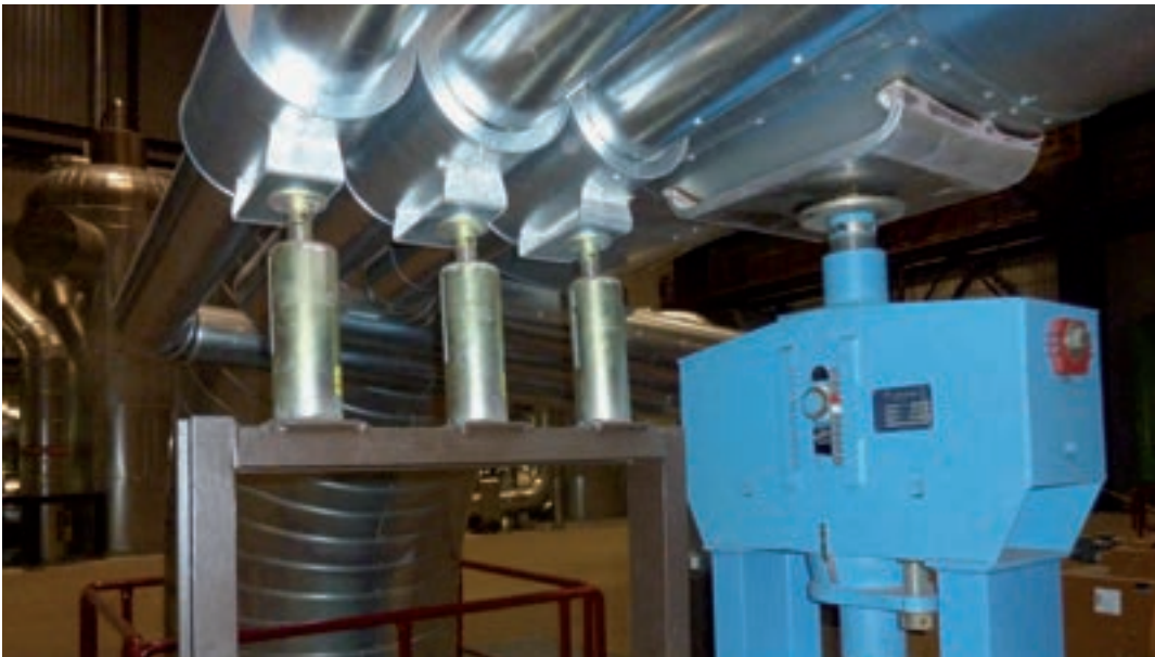
Typical use of slide plates under clamp bases
