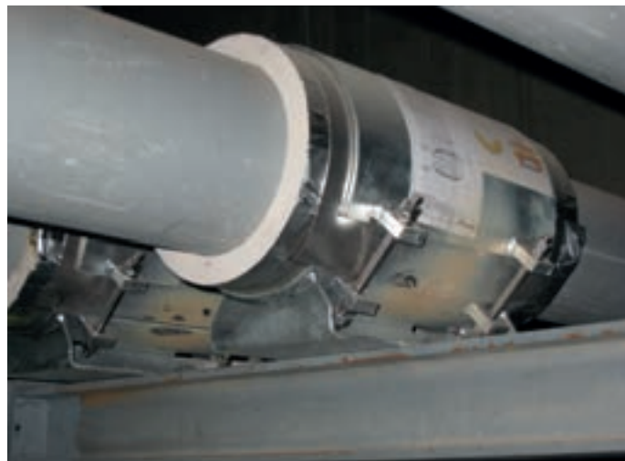
Cryogenic clamp base type 56
