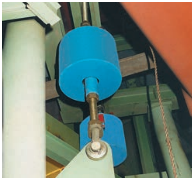
Spring hanger type 22 with threaded clevis type 61 mounted
