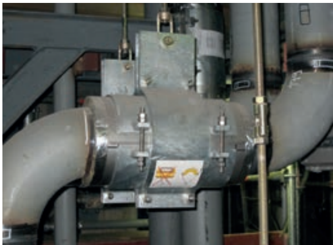
Suspension with cryogenic pipe clamps
