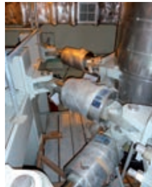
Securing pipe systems with snubbers type 30
