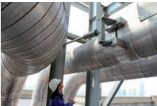
Inspection of supports at the plant
