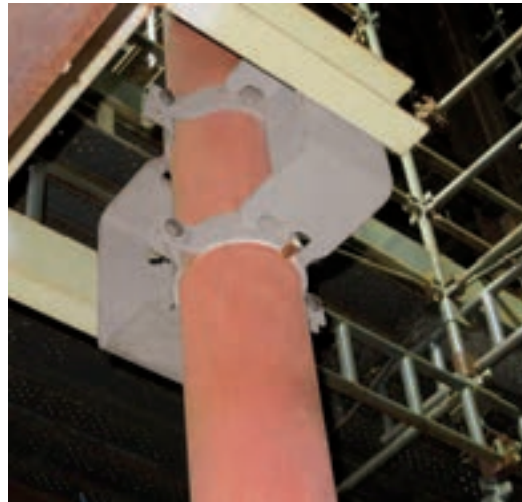
Pipe bearing (type 49 ... G2P)
