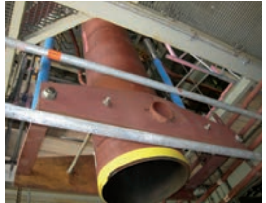
Type 34 with snubbers and position-securing devices
