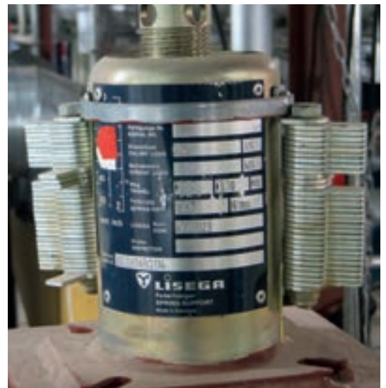
Type 29 with blocking devices attached
