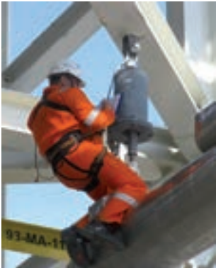
Controlling a pipe support
