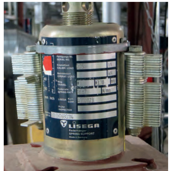
Type 29 with blocking devices attached
