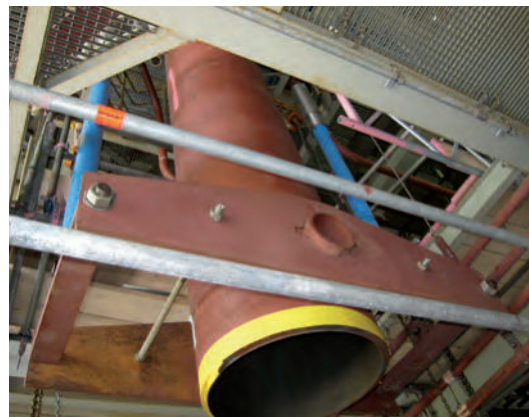
Type 34 with snubbers and position-securing devices
