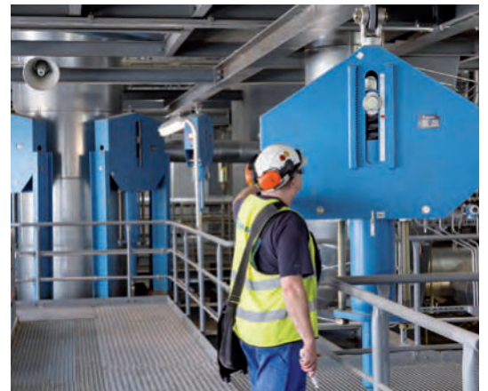
Installation inspection of a constant hanger
