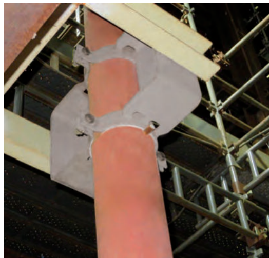
Pipe bearing (type 49 ... G2P)
