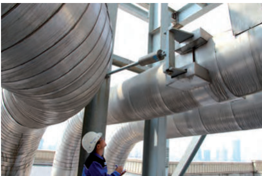
Inspection of supports at the plant
