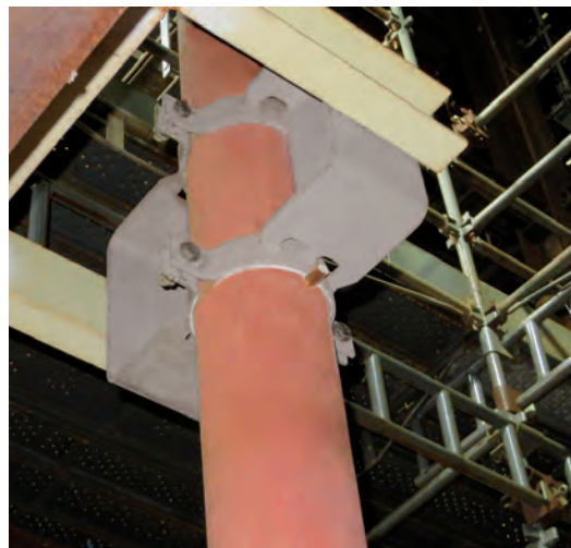
Pipe bearing (type 49 ... G2P)
