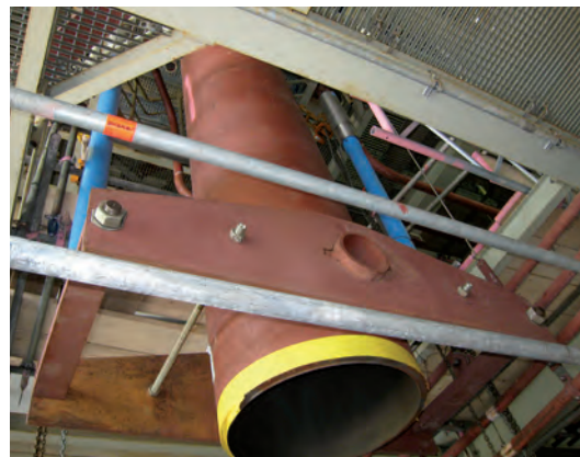
Type 34 with snubbers and position-securing devices
