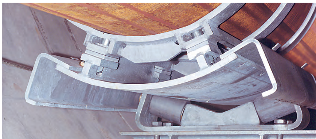
Special pipe saddle type 54 with double cylinder roller bearing type 53 and lift-off restraints type 55
