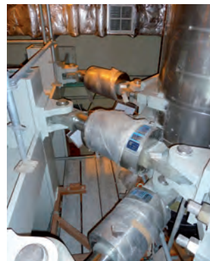
Securing pipe systems with snubbers type 30
