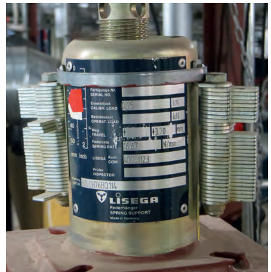
Type 29 with blocking devices attached
