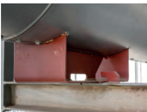
Lift-off restraint
