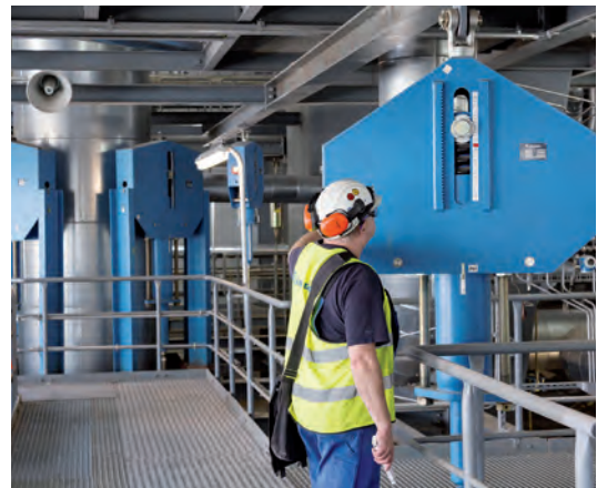
Installation inspection of a constant hanger
