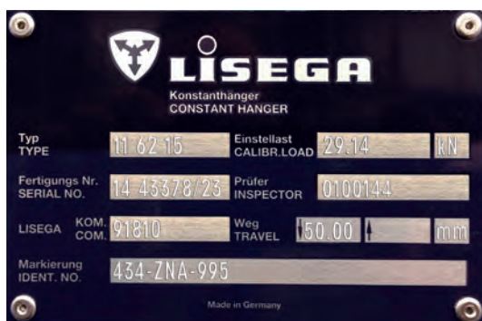
Name plate with stamped operating data
