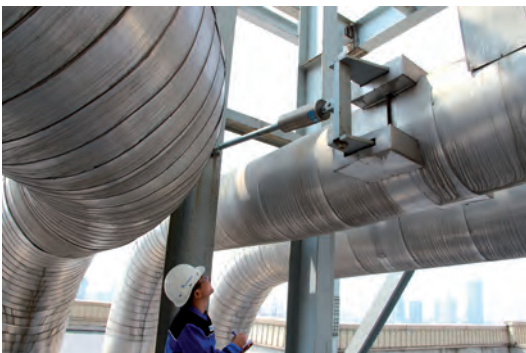
Inspection of supports at the plant
