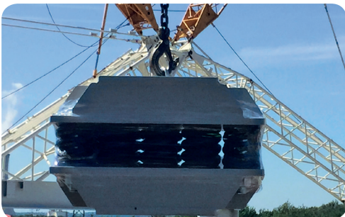
Fig. 3 Lifting of spring element with eye bolt
