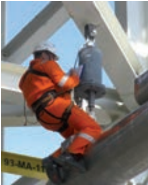
Controlling a pipe support
