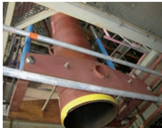
Type 34 with snubbers and position-securing devices
