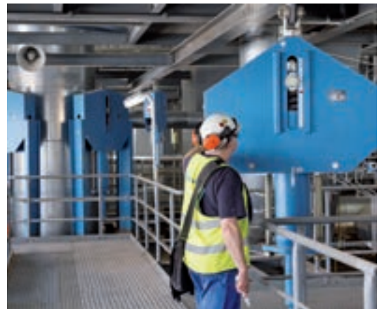
Installation inspection of a constant hanger
