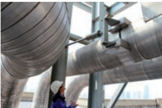
Inspection of supports at the plant
