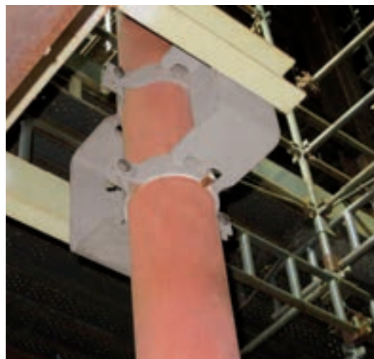
Pipe bearing (type 49 ... G2P)
