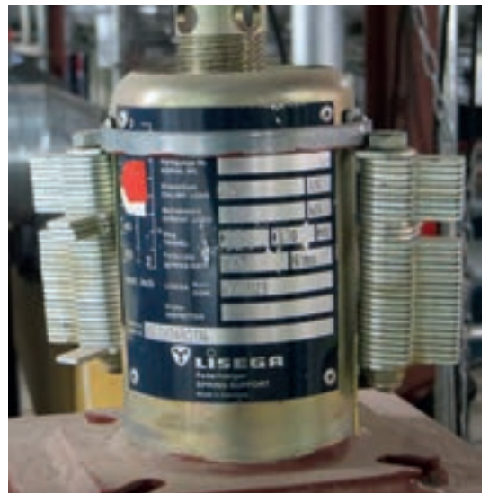
Type 29 with blocking devices attached
