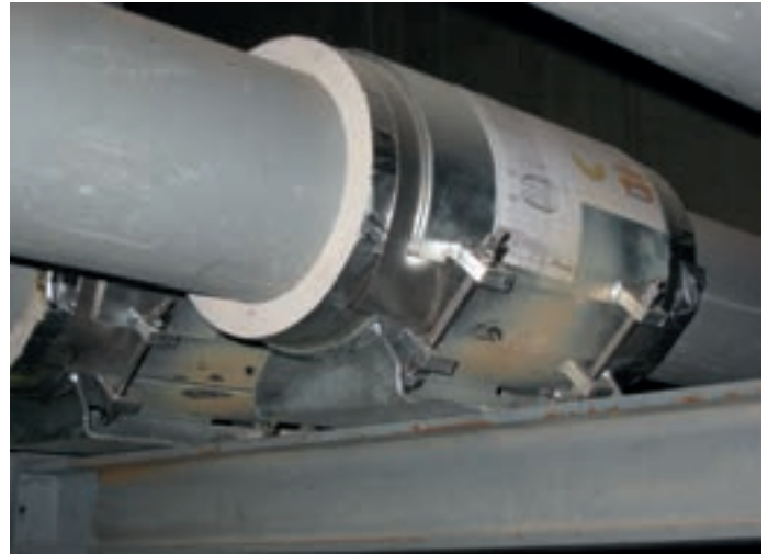
Cryogenic clamp base type 56
