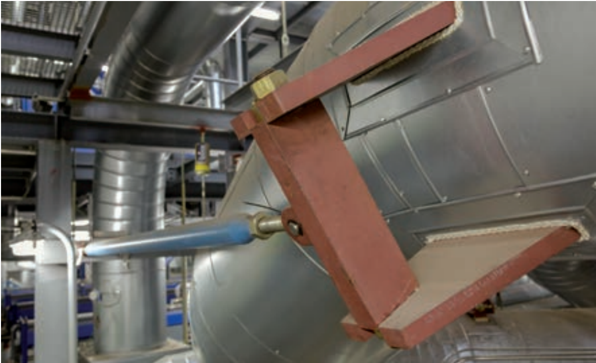
Horizontal axial stop with rigid struts type 39 and pipe clamp type 34
