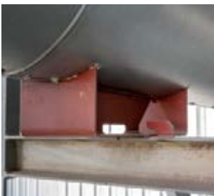
Lift-off restraint
