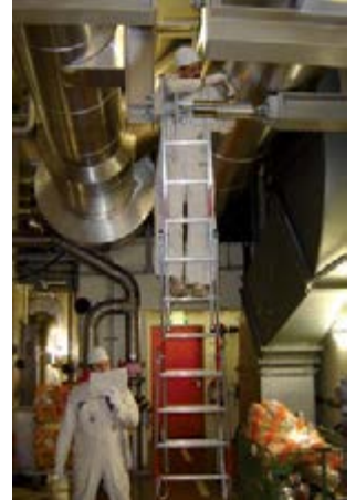
Visual inspection of snubbers
