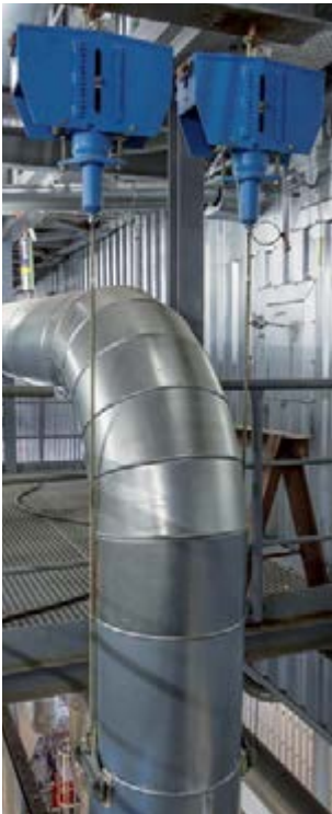
Constant hanger in a coal-fired power station
