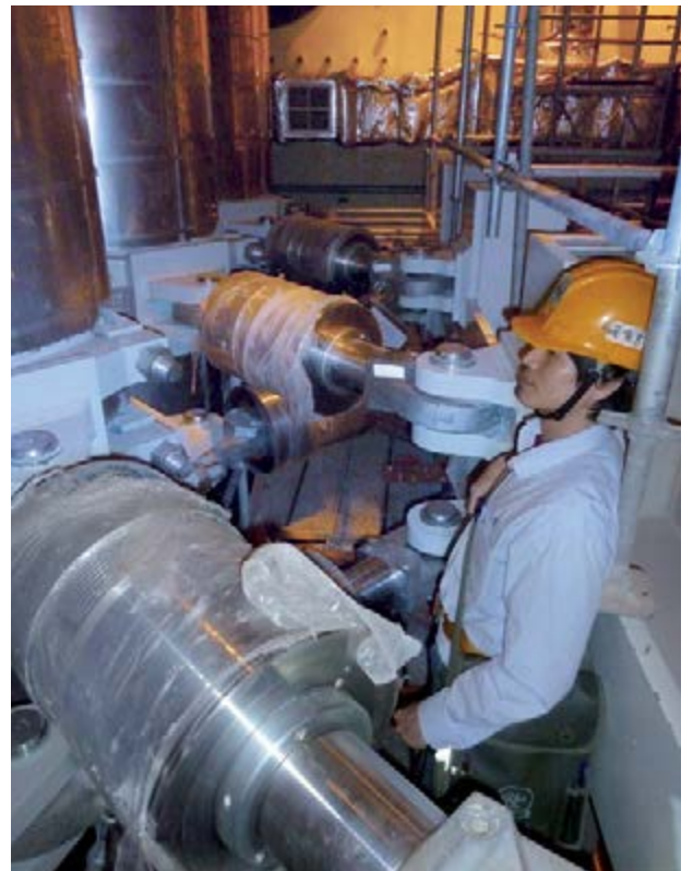
Commissioning of type 30
