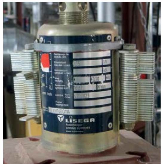
Type 29 with blocking devices attached
