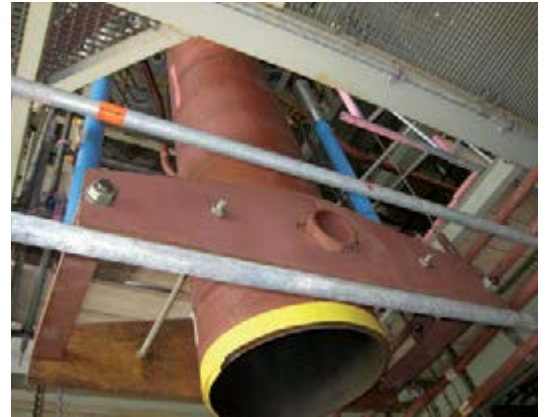
Type 34 with snubbers and position-securing devices
