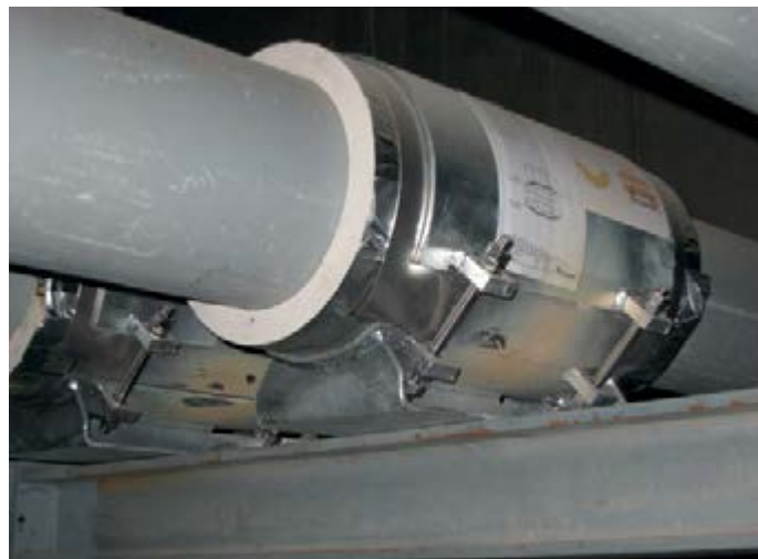
Cryogenic clamp base type 56
