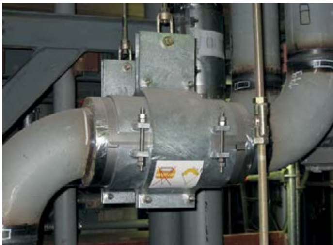
Suspension with cryogenic pipe clamps
