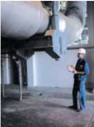
Check on correct installation
